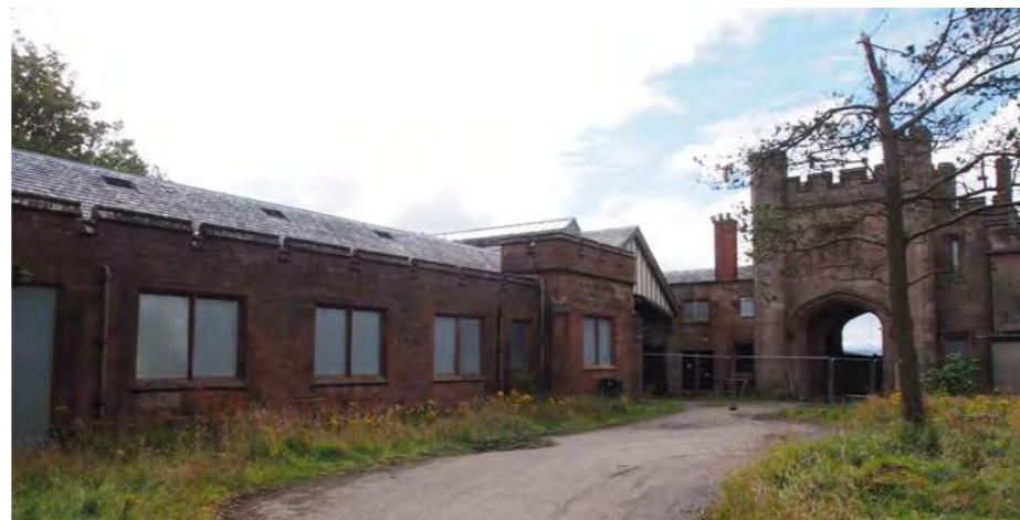
Gate House rear elevation
