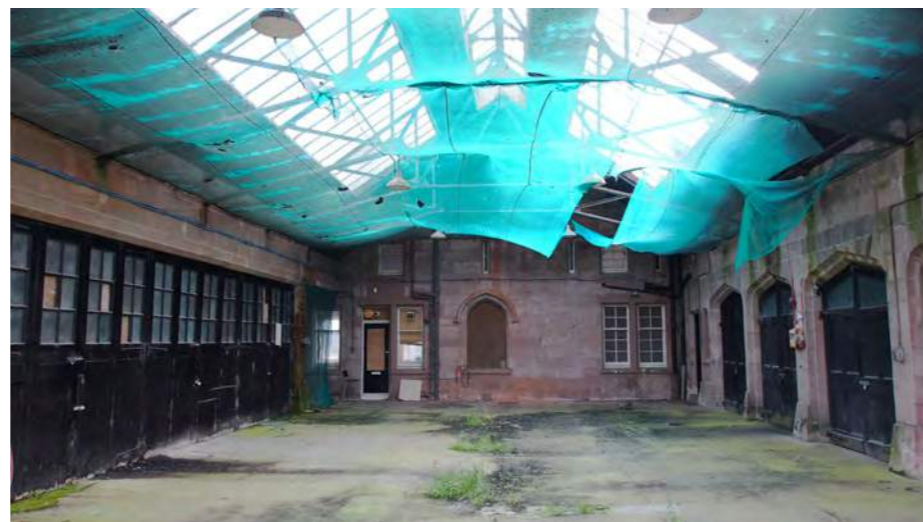
Gate House covered yard
