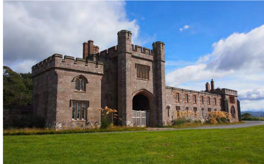
Gate House main elevation
