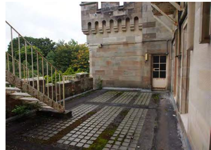
First Floor West Balcony
