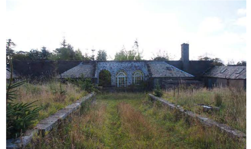
Greenhouse and workshop
